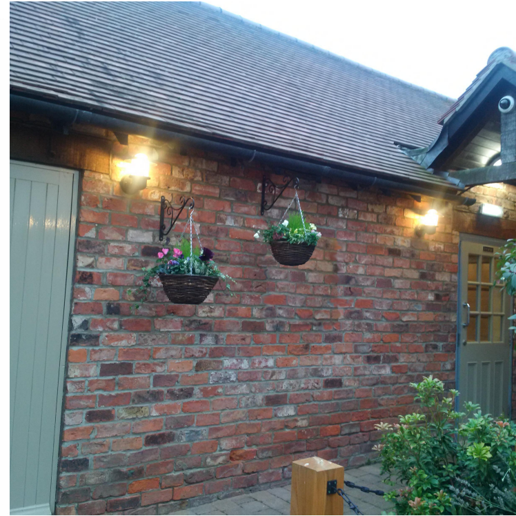
PHOTOGRAPH OF PROPOSED BRICKWORK AND ROOF TILING
